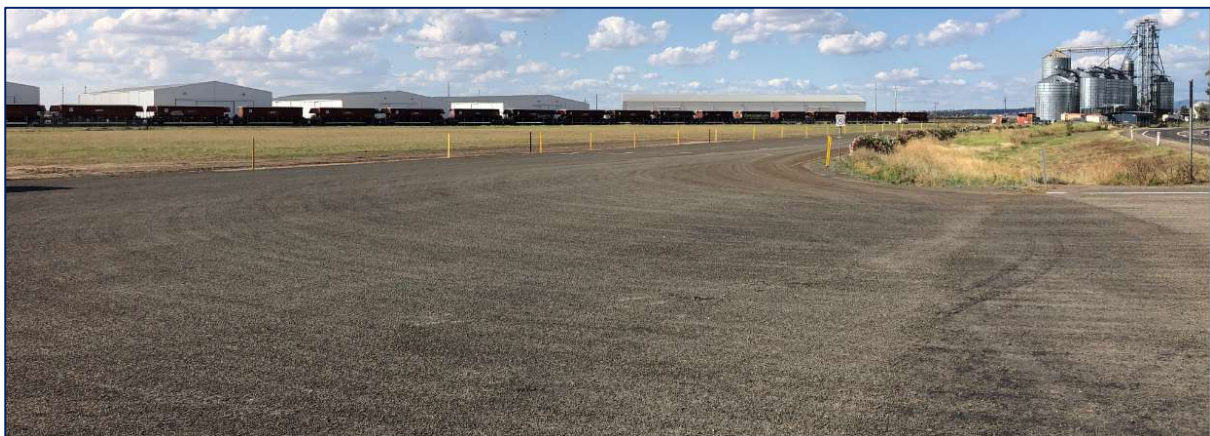
Figure 1: Recently sealed and widened bitumen access road to the weighbridge and office at Arrow Commodities grain receival terminal in Narrabri
